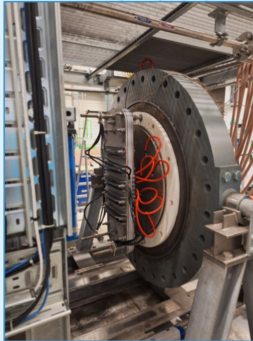
BTU test site with the short stack and pressure vessel, Source: PEACE project (CC-BY-NC-ND 4.0)
